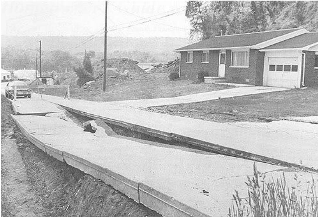
Figure 4. Cracked and dislocated street across an old slide resulted from soil movement under weight. House is now endangered. (Photo by USDA-Natural Resources Conservation Service)
