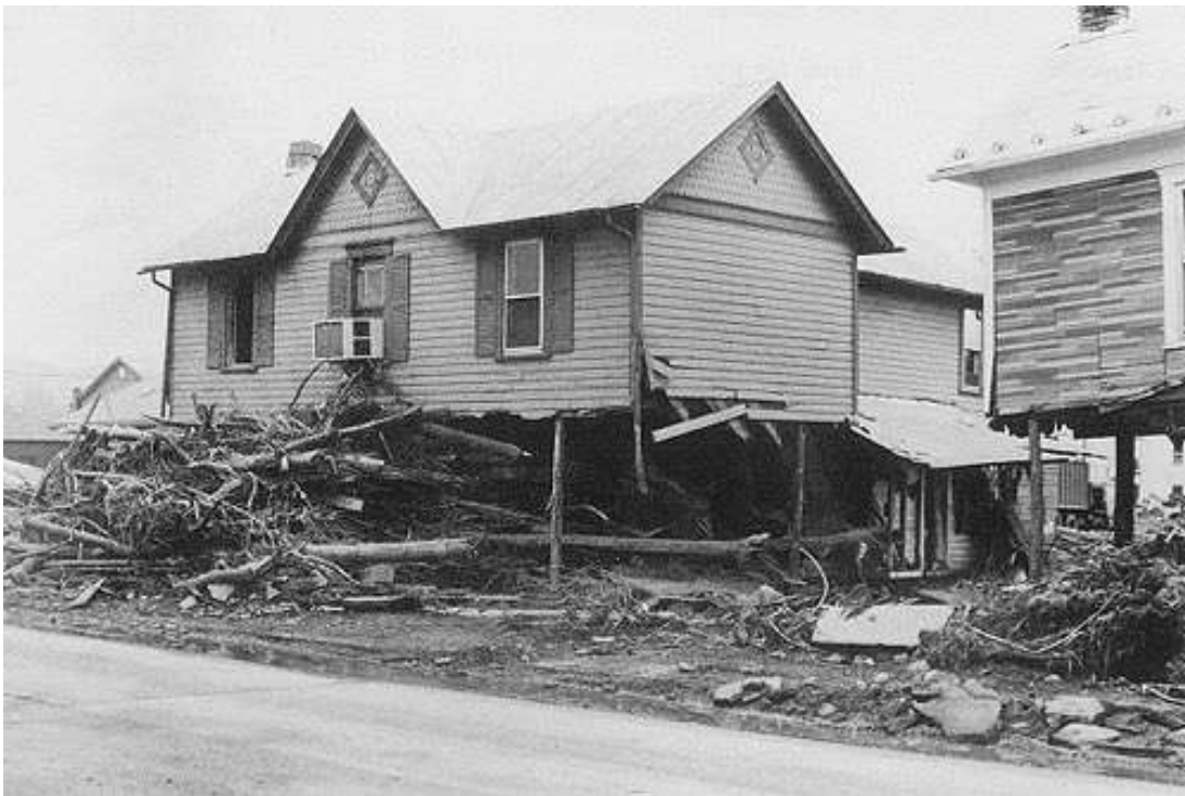
Figure 1. Destroyed houses in Petersburg, Grant County, are casualties of the November 1985 flood. (Photo by Peter Lessing)
