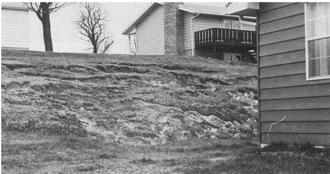
Figure 3. Slump and earthflow in a new housing development. (Photo by Peter Lessing)
