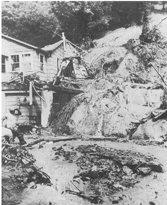
Figure 5. July 1973 landslide in Kanawha City, Kanawha County. (Photo courtesy of the Charleston Gazette)
